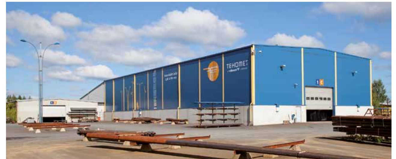
Tehomet decorative steel poles production in Kangasniemi.
