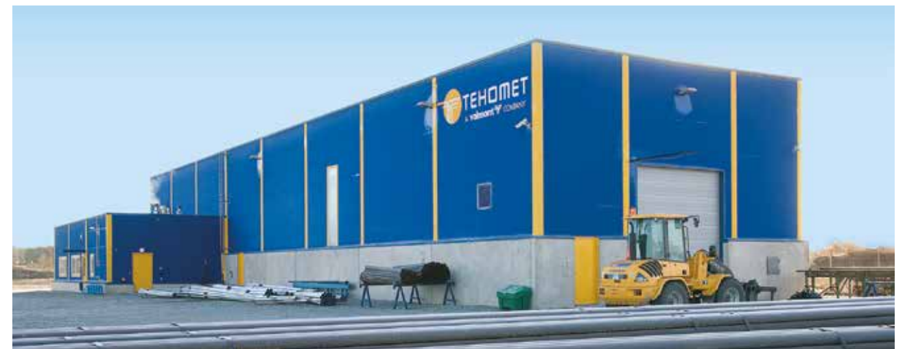
Steel poles production in Kiiu, Estonia.
